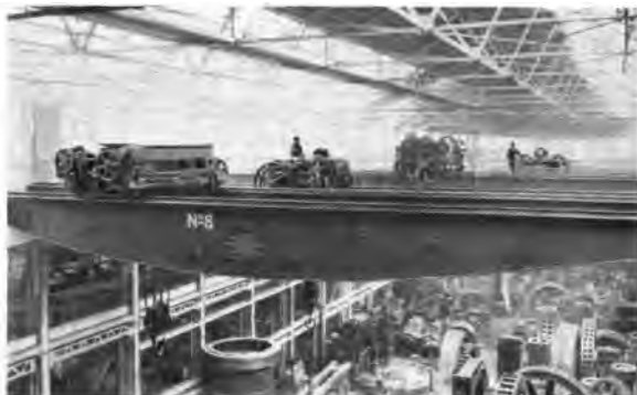
Four of the Cranes in Section B, Westinghouse Electric & Mfg. Co.
